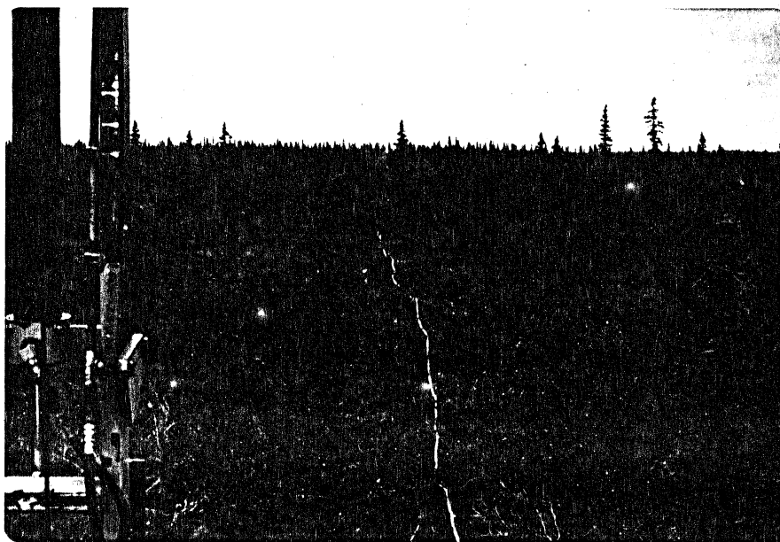
Drilling test hole 19 - view looking northeast along proposed alignment 7/23/73 D.P.
