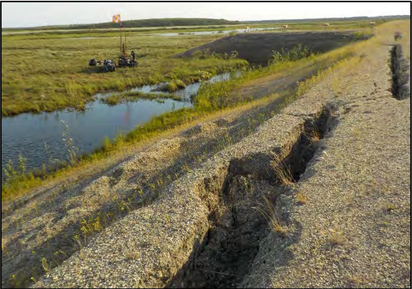
Figure 4. Shoulder cracks and ponding looking southwest at the PAPI and TH19-3030.
